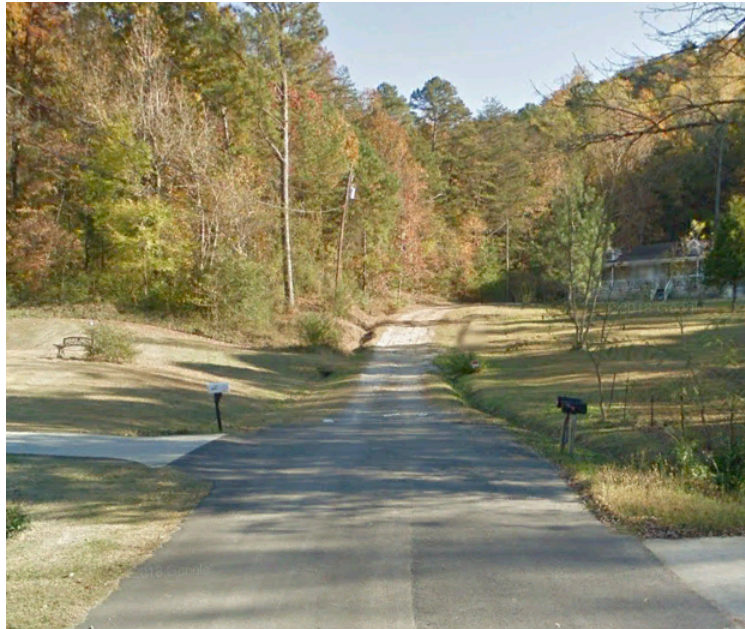
Existing Private Drive
